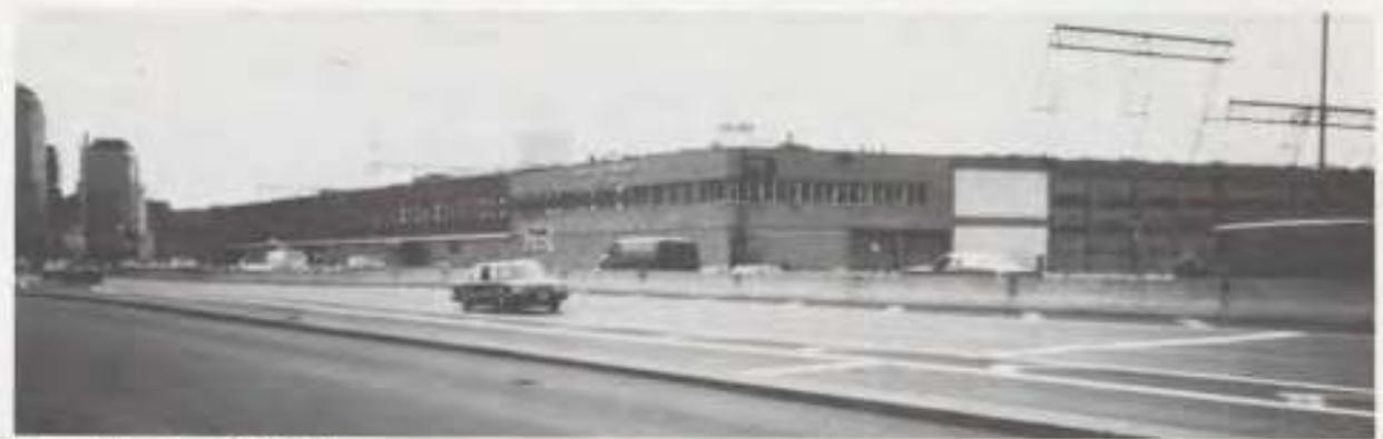
The existing face of Pier 40.
